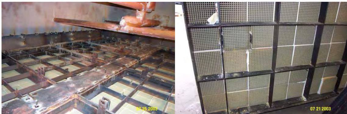
**Figure 5:** Installation of the first catalyst layer – July 2003
