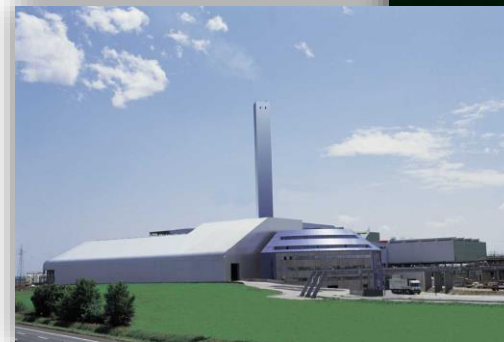
Brescia Waste-to-Energy plant, Italy
