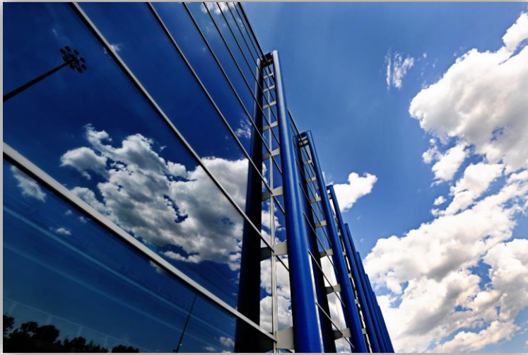
Torino Waste-to-Energy plant, Italy
