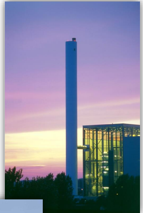
Malmö Waste-to-Energy plant, Sweden
