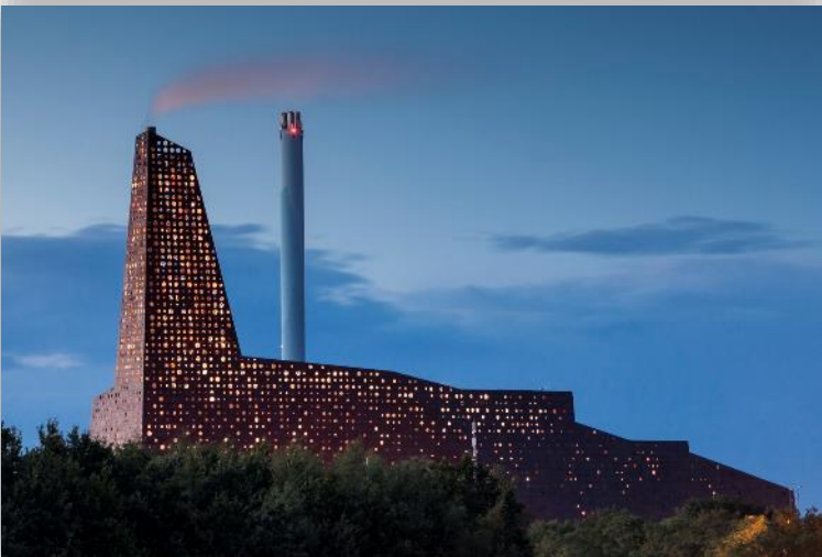
Karanoveren Waste-to-Energy plant, Denmark
