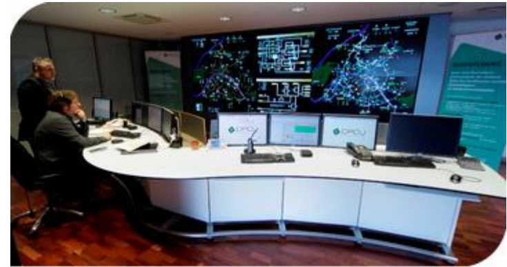
The CPCU dispatching centre was entirely re-engineered in 2010. It is a world first for such a large network.
