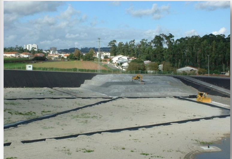
Specific landfill – for inert ashes disposal
