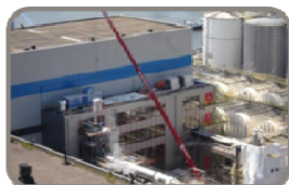
Waste incinerator and energy plant
