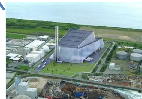
Dublin WtE Facility, Eastern-Midlands Region
