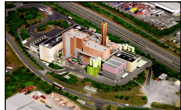
The waste-to-energy plant in 2012.
