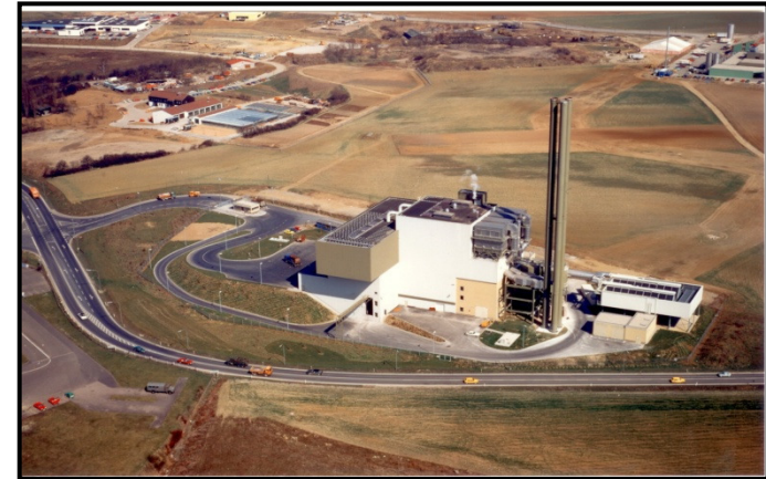
The waste-to-energy plant in 1984.
