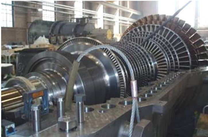
turbine MVA Bielefeld
