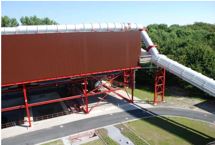
Air condenser MVA Bielefeld
