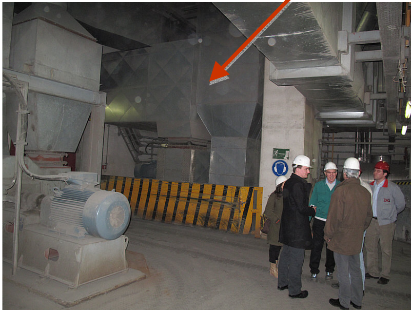
Integration into the secondary air duct
