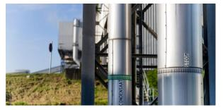
for thousands of tonnes of CO<sub>2</sub> emissions. ECLUSE is a collaborative project to deliver steam from local WtE plants to six industrial companies through a high-pressure pipeline. The project which came online in 2019 replaces fossilbased energy with steam from WtE, improving the efficiency of the WtE plants and ensuring a cost-effective and long-term energy supply for neighbouring industries.
