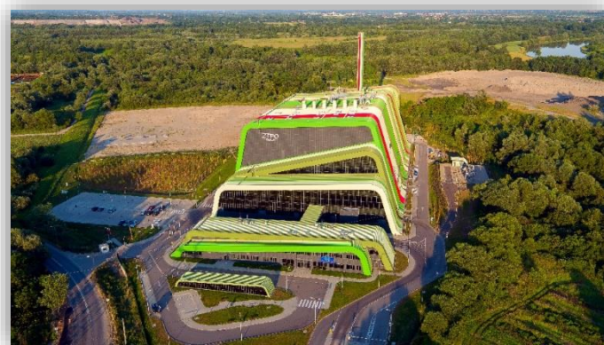
Krakow WtE plant, Poland
