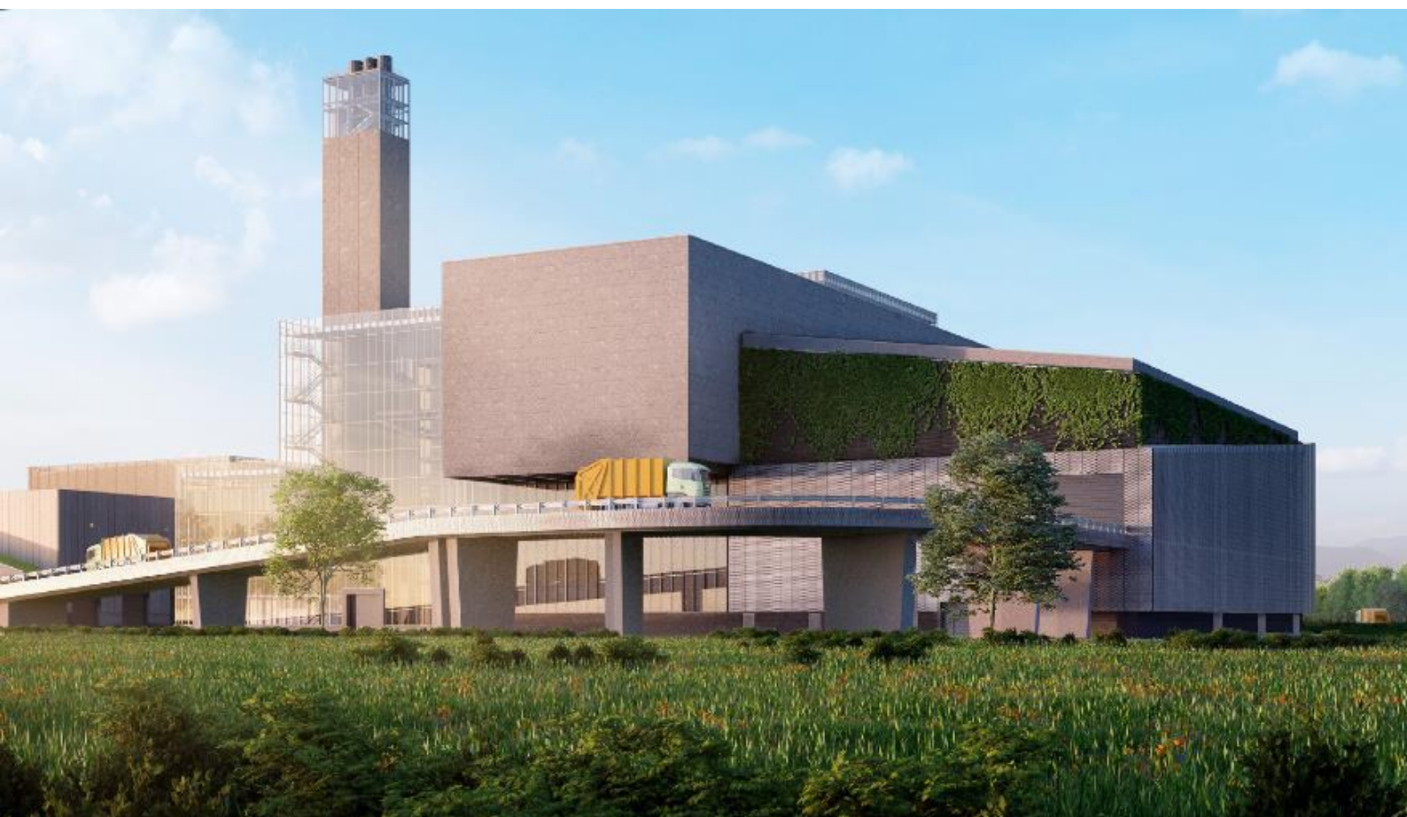
Planned WtE plant in Warsaw, source: MPO Sp. z o.o. w m.st. Warszawie. Image by courtesy of Doosan Lentjes GmbH.
