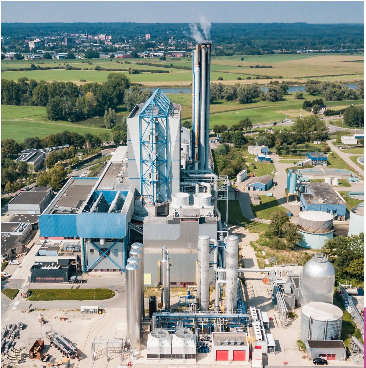
AVR WtE Plant (back) and CO 2 capture Unit (front), Duiven - The Netherlands. © AVR Afvalverwerking B.V.
